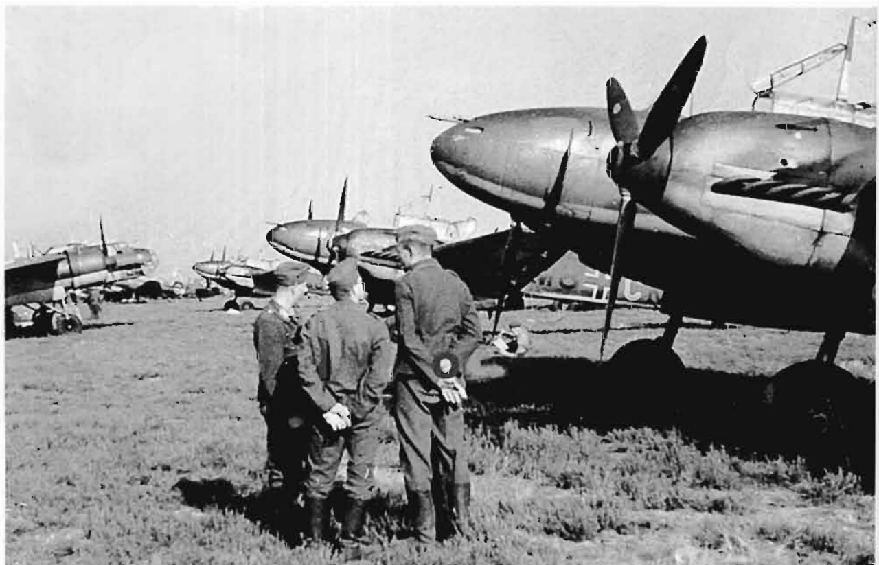
ABOVE: A Bf 110 C-1 of I./ZG 76. Note the two antennae extending from the cockpit mast. The spinner tip and the aircraft letter 'B' on the nose would appear to be in yellow, making this a 3. Staffel machine. The emblem is not identified, but appears to be a figure of a bird standing at the top of northern Europe, not dissimilar to the emblem used by JG 1 when it was based in that locality.
